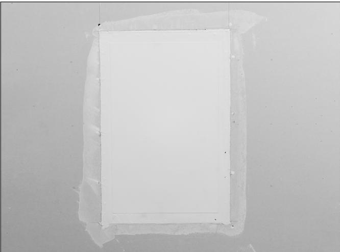
4. Place mesh tape over the drywall seams. Overlap tape slightly.
