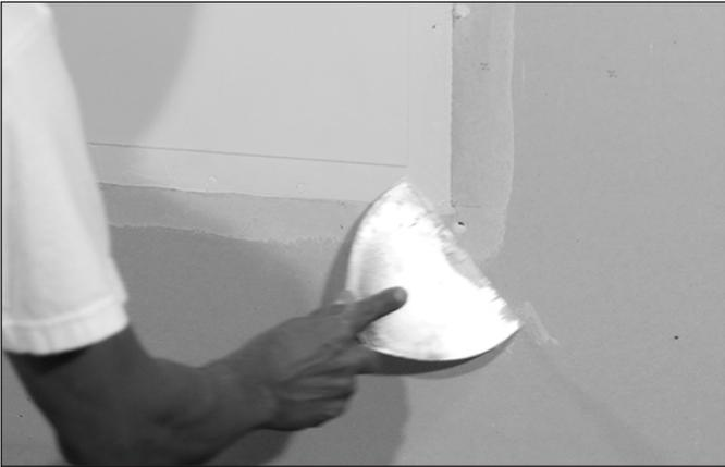
3. Allow hot mud to set slightly before applying mesh tape.
