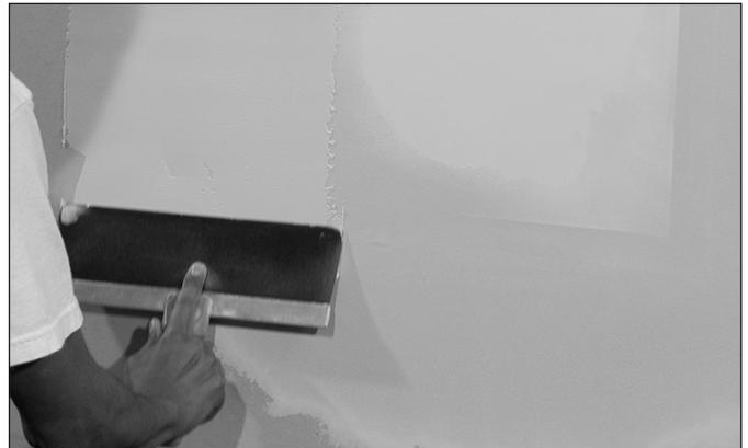
11. Compound buildup on the active surface of the speaker should not exceed 1/16" (1.5mm).
