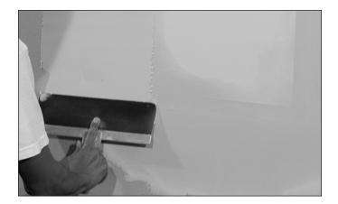
11. Compound buildup on the active surface of the speaker should not exceed 3mm (1/8").
