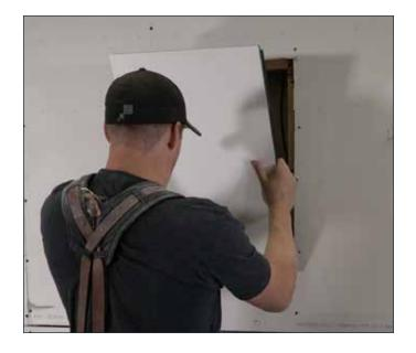
12. Ensure the center of the speaker diaphragm (not the recessed edges) is flush with the surrounding drywall. Adjust shims if necessary.
